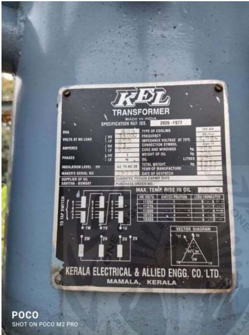
Name plate details of transformer
